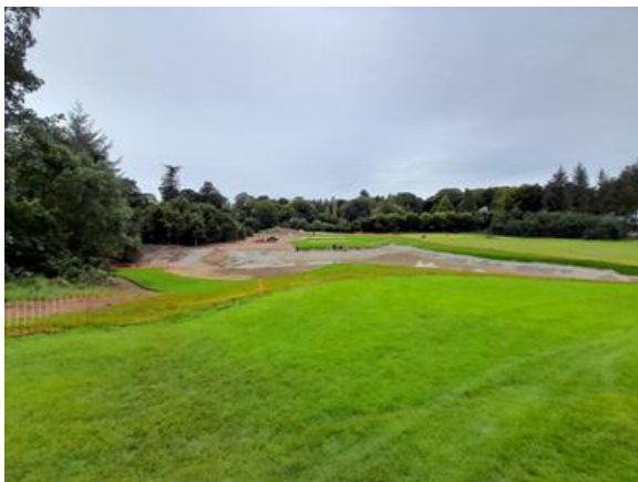
Image 30 Lake 2 near completion
