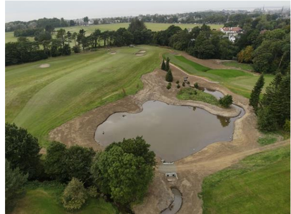
Image 29 Aerial view of new lake 1
