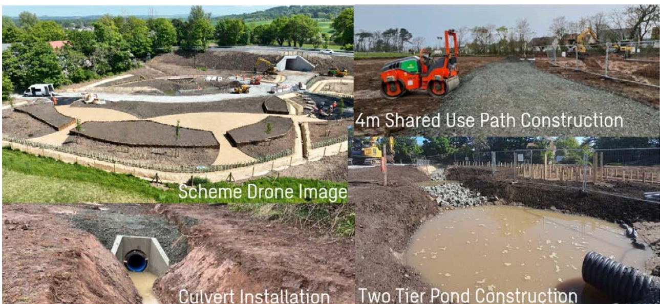
Figure 0-2 Photo collage showing different elements of the construction phase
