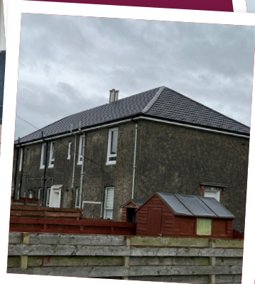
Replacement Roof Covering, Ayr
