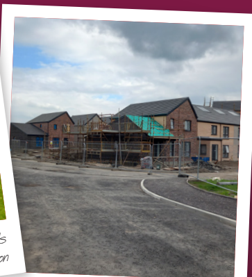
New Build Housing Development under construction at Mainholm, Ayr.
