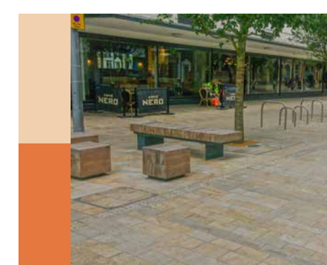
1 Slabbed Footways & Crossovers Material: Granite Origin - Portugal Colour - Lustre Leve Multi Finish - Flamed
