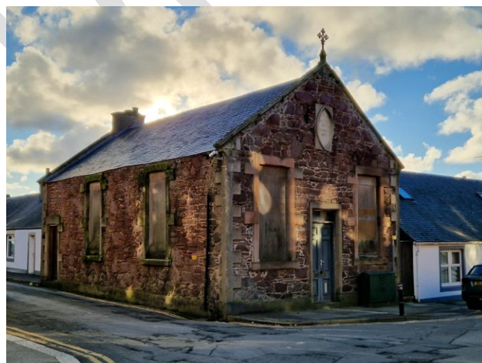
Former Methodist Chapel, Wilson Street
