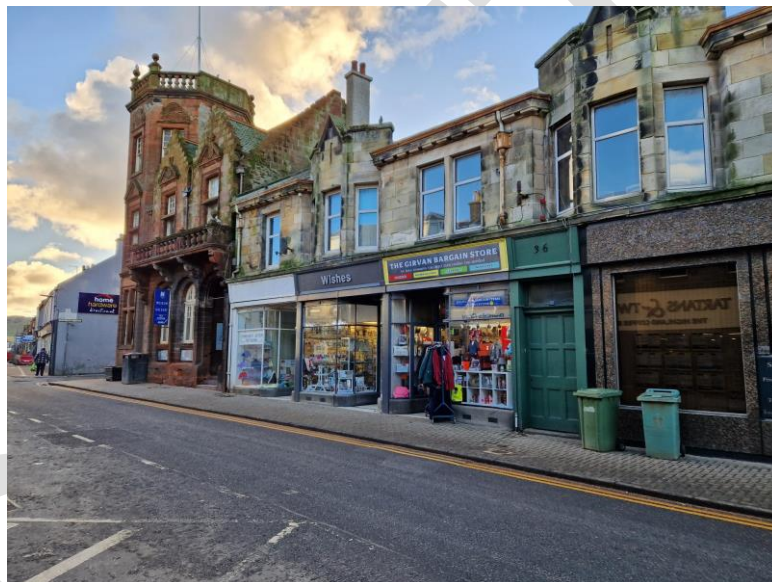
Traditional Shopfronts, Dalrymple Street
