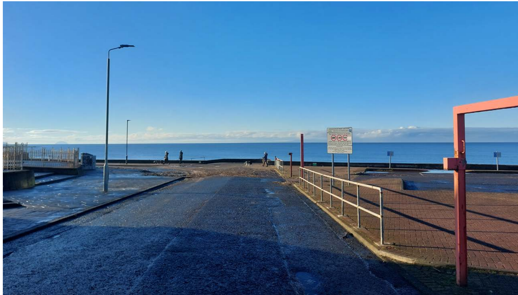
Promenade at Grangemuir Road - Current Condition
