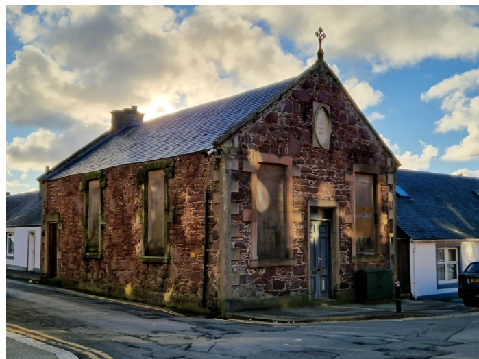
Former Methodist Chapel, Wilson Street
