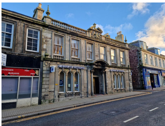
Stonework Erosion, 17 Dalrymple Street
