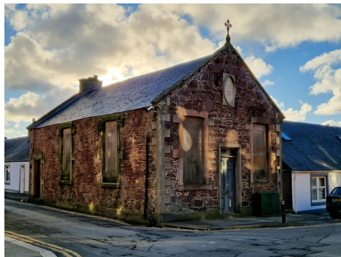
Former Methodist Chapel, Wilson Street
