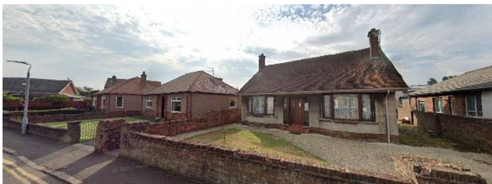
Photo No 3 (St Quivox Road looking East)
