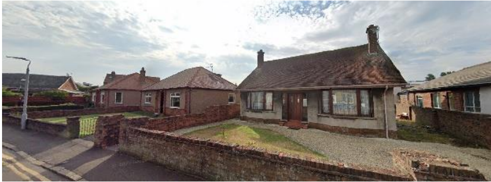
Photo No 3 (St Quivox Road looking East)
