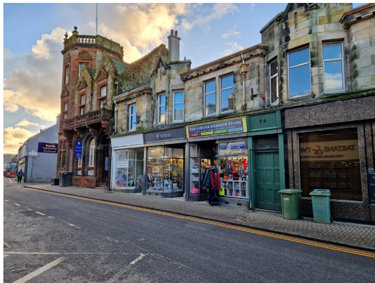
Traditional Shopfronts, Dalrymple Street
