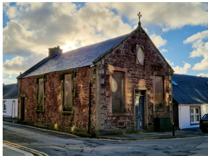
Former Methodist Chapel, Wilson Street
