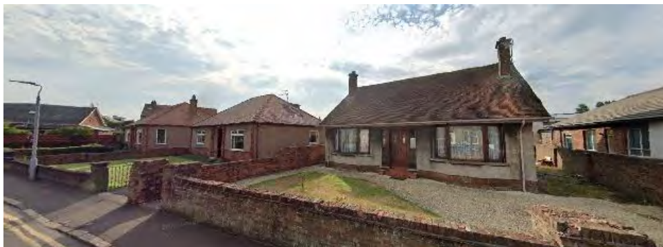
Photo No 3 (St Quivox Road looking East)
