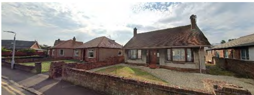
Photo No 3 (St Quivox Road looking East)
