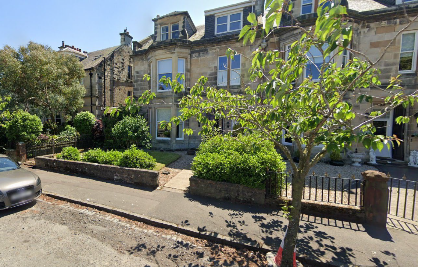
Fig. 6 - Existing wall at 38 Park Circus and neighbouring front garden with hard landscaping.
