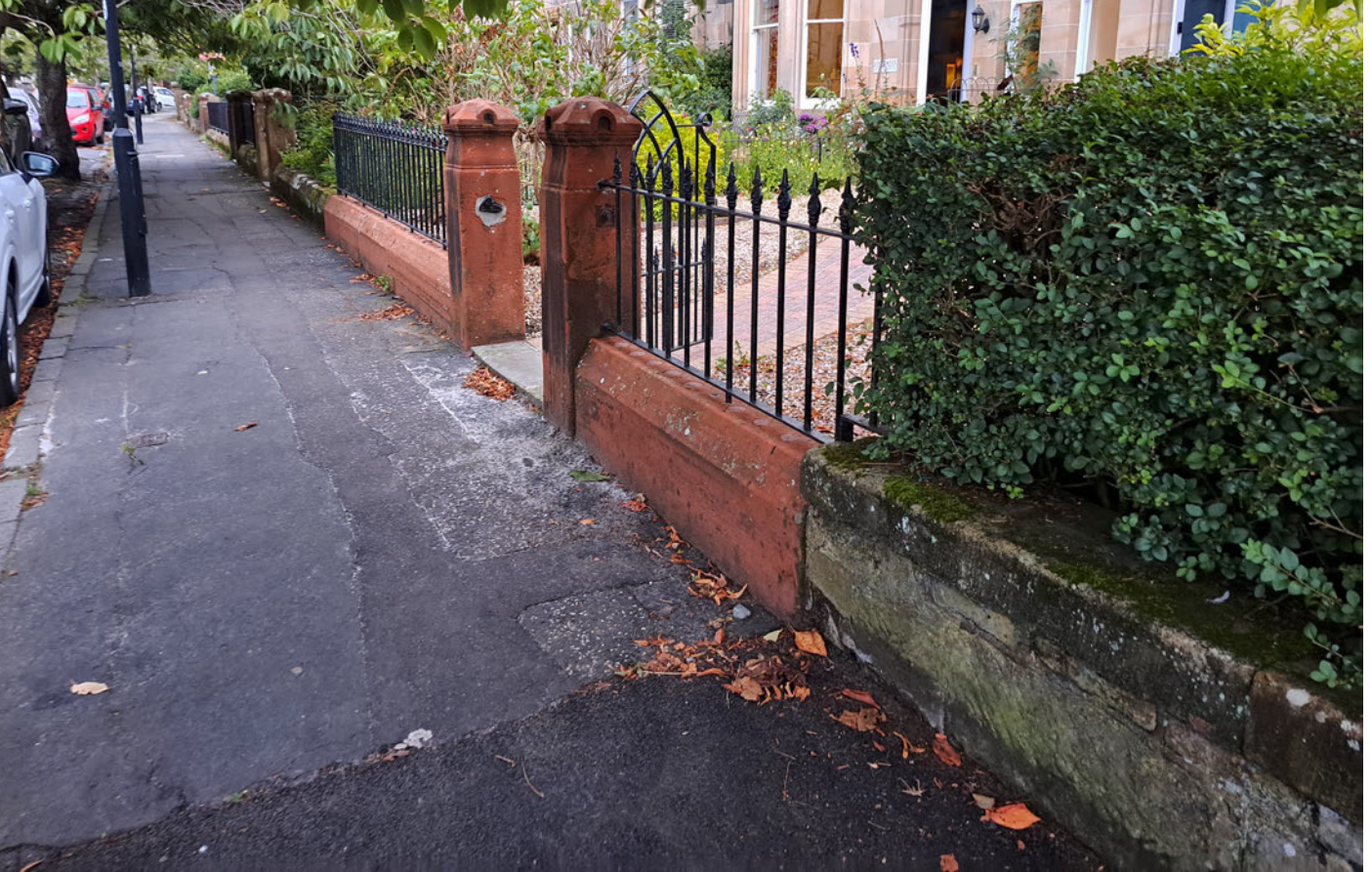
Fig. 8 - Change of materiality, form, height and treatment above the wall between 28 and 30 Park Circus.
