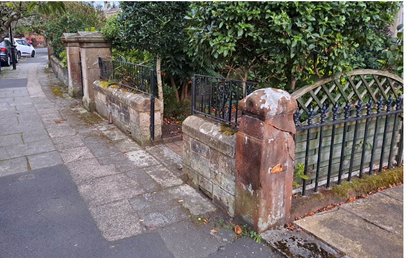
Fig. 7 - Change of materiality, height and treatment above the wall from 38 and 40 Park Circus.
