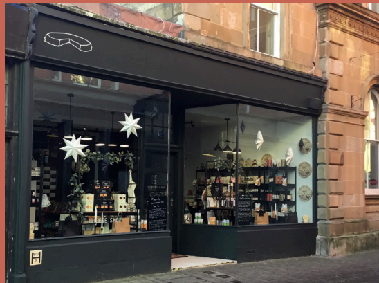
Effectively restrained shopfront at 71 Newmarket Street
