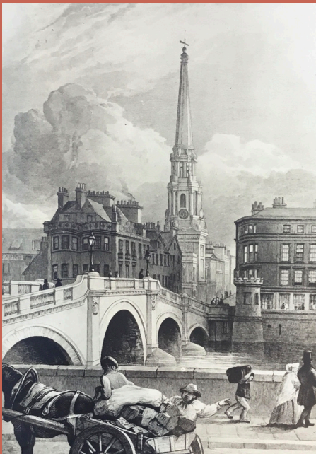
Former New Bridge and Steeple © Ayrshire Archives
