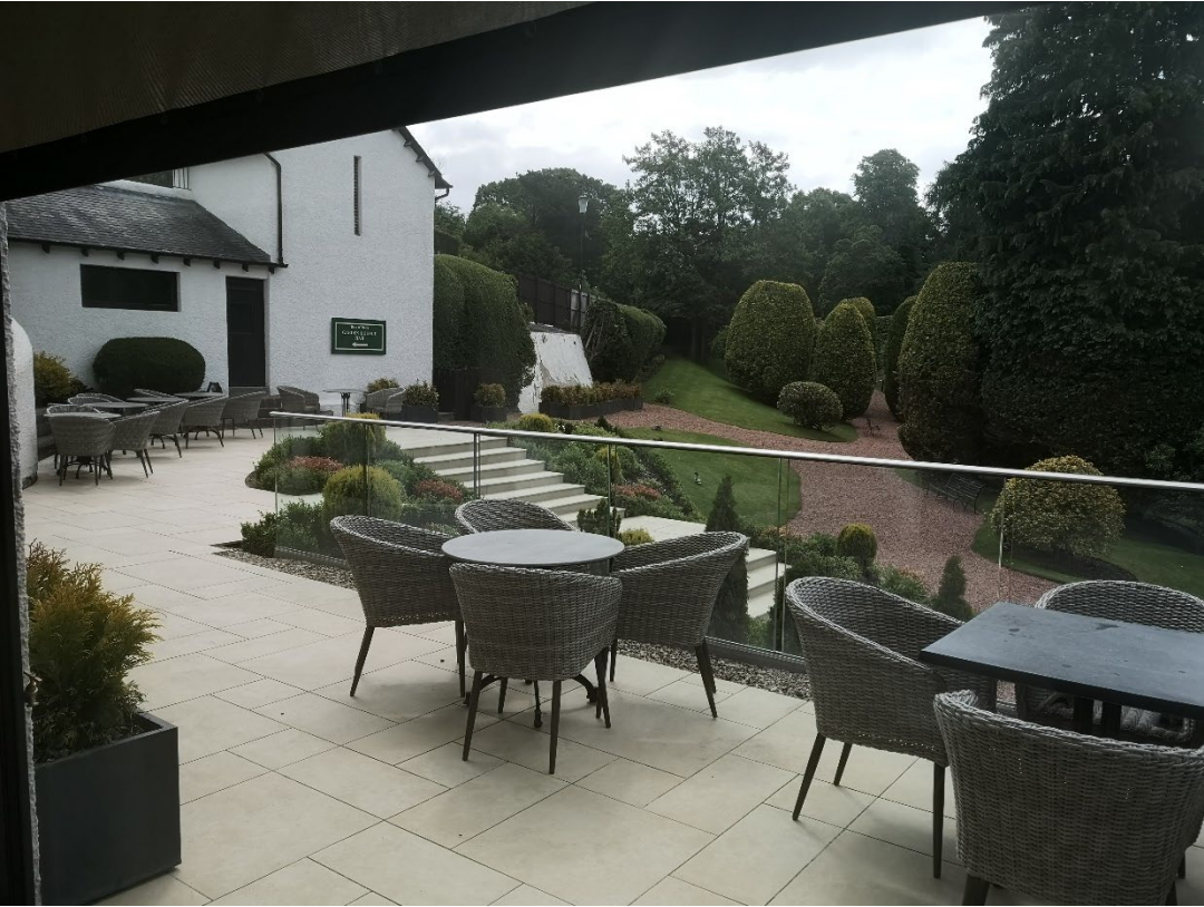
Newly formed balcony/terrace outside the pre-function area
