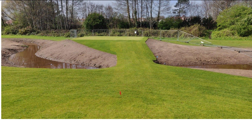
Figure 3 New 2nd Green and Drainage Ditches
