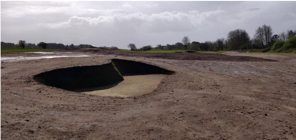
Figure 2 Reprofiled Fairway during construction
