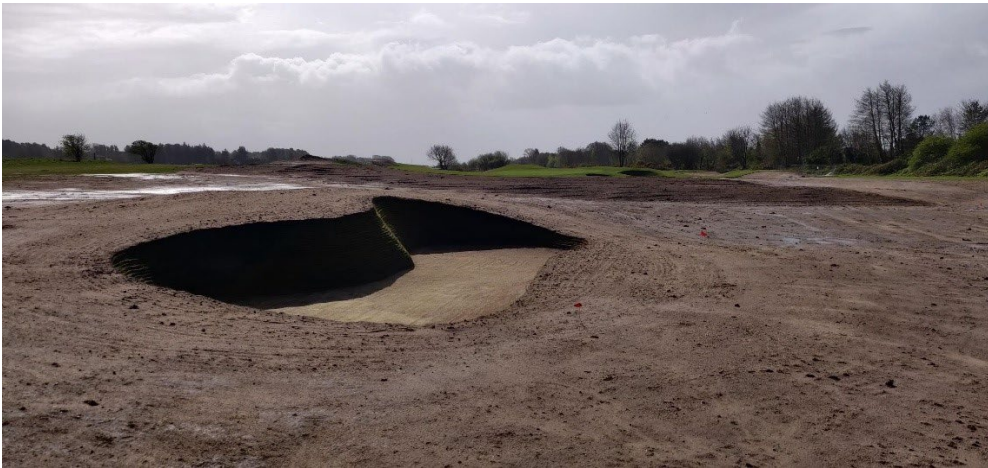
Figure 2 Reprofiled Fairway during construction
