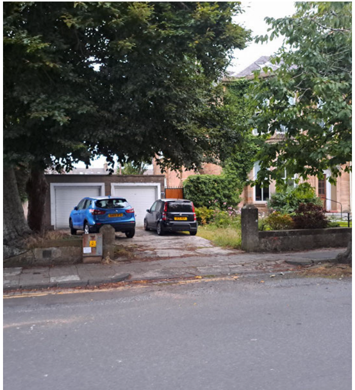
Fig. 14 - 3 Park Circus drive entrance at end of terrace.
