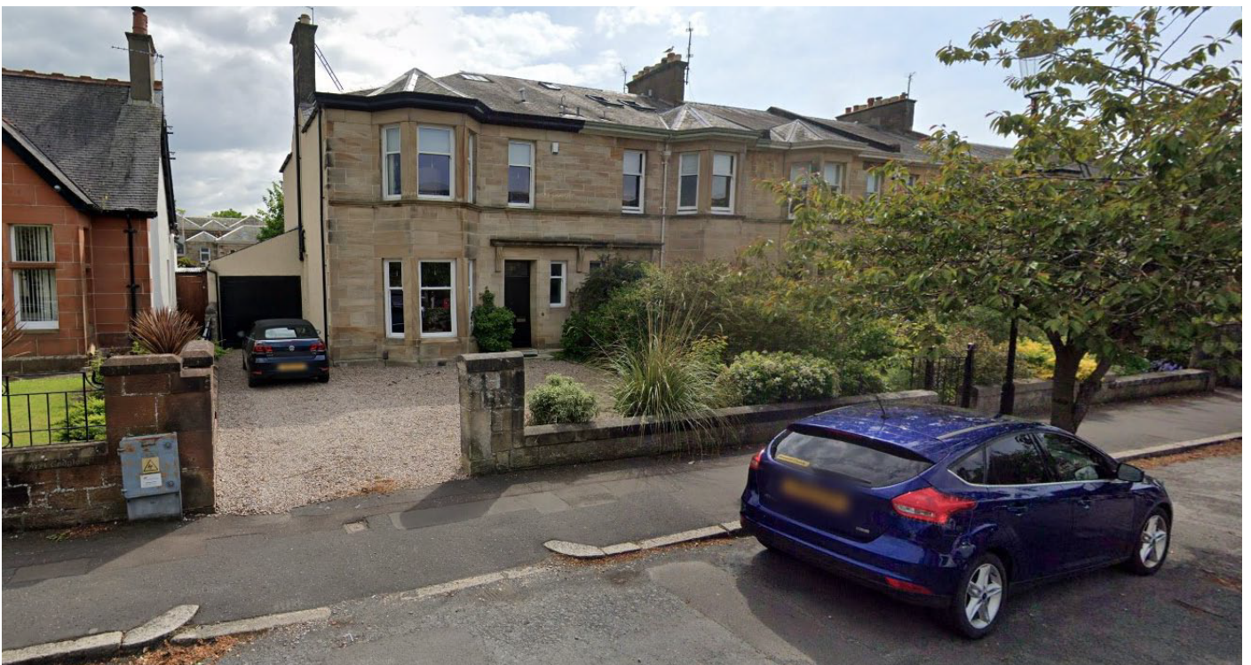
Fig. 11 - 27 Bellevue Crescent drive entrance at end of uniform terrace.
