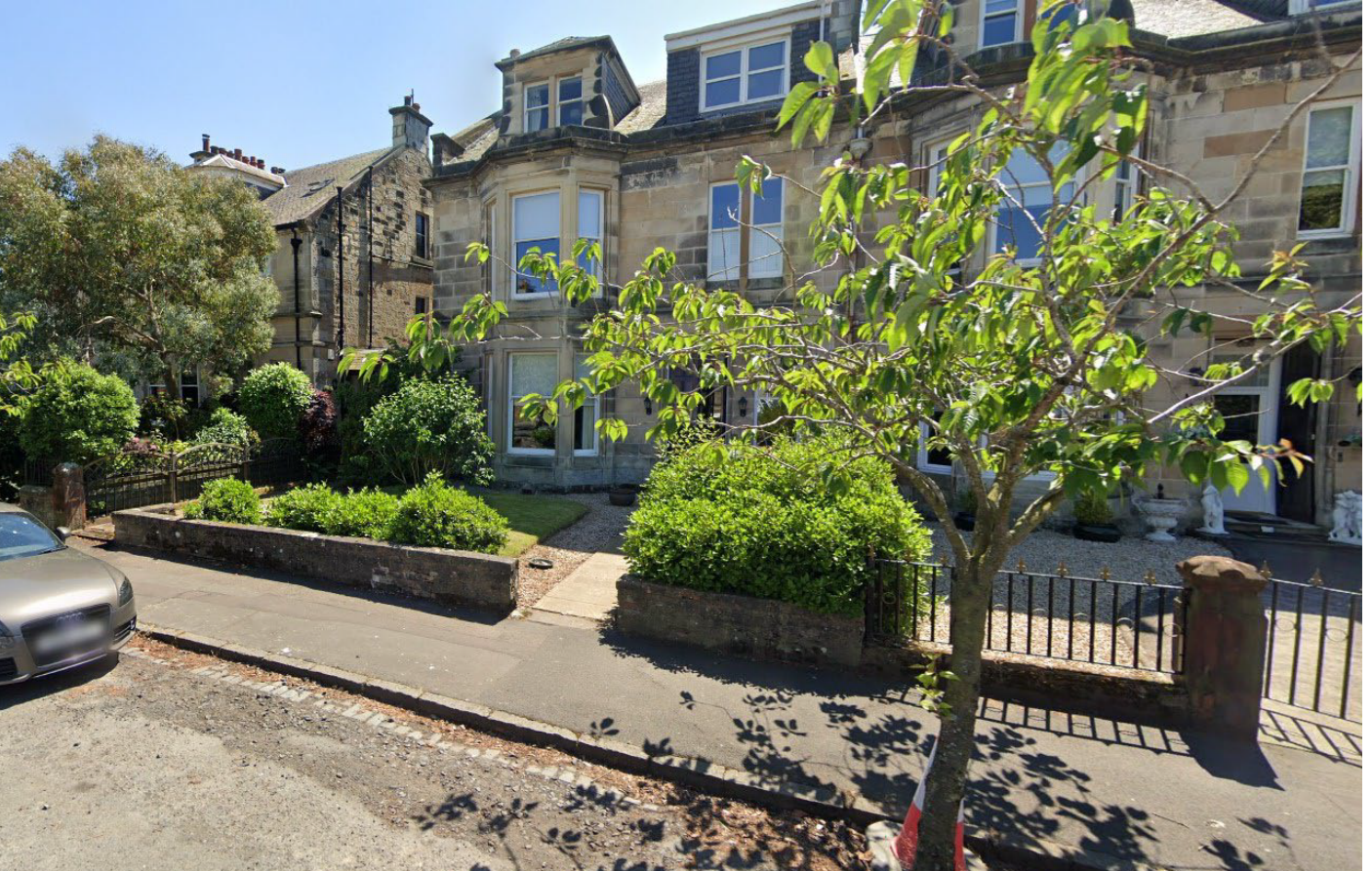
Fig. 6 - Existing wall at 38 Park Circus and neighbouring front garden with hard landscaping.
