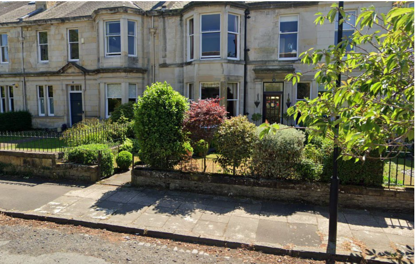
Fig. 9 - Change of materiality, sandstone size, height and treatment above the wall between 22, 24 and 26 Park Circus.
