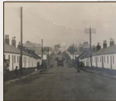
UNIFORMED TERRACED MINERS' COTTAGES, WITH COAL HEATING AND STREET TELEGRAPH POLES
