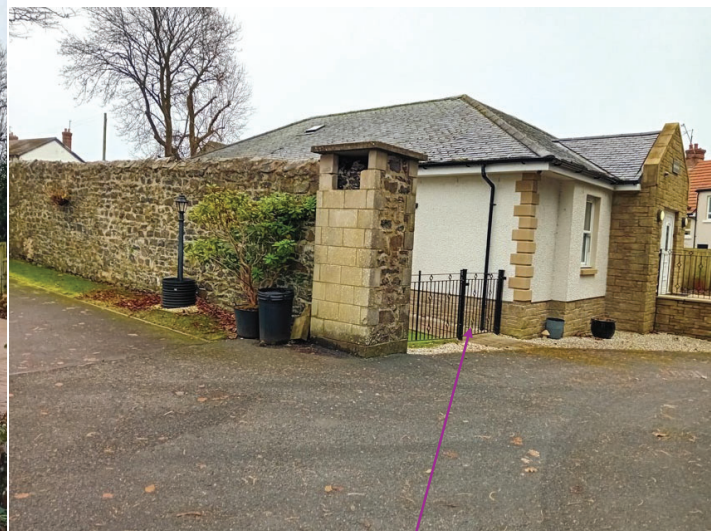
Access to proposed house. Photo taken from front garden of No.64 Main Street sandwiched between donor property.
