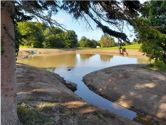
Image 28 New lake 1- overflow from Slaphouse at culvert on far left
