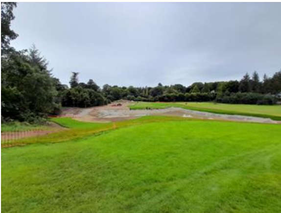
Image 30 Lake 2 near completion
