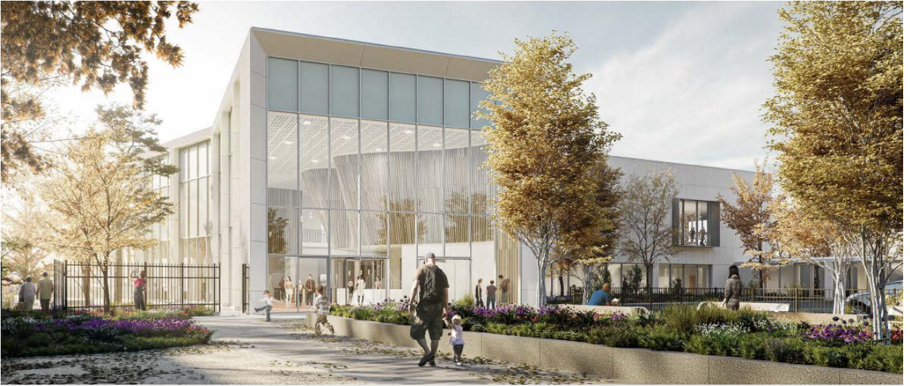
Front Entrance from Alloway Street
