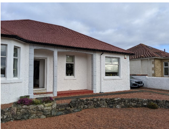
view towards front entrance
