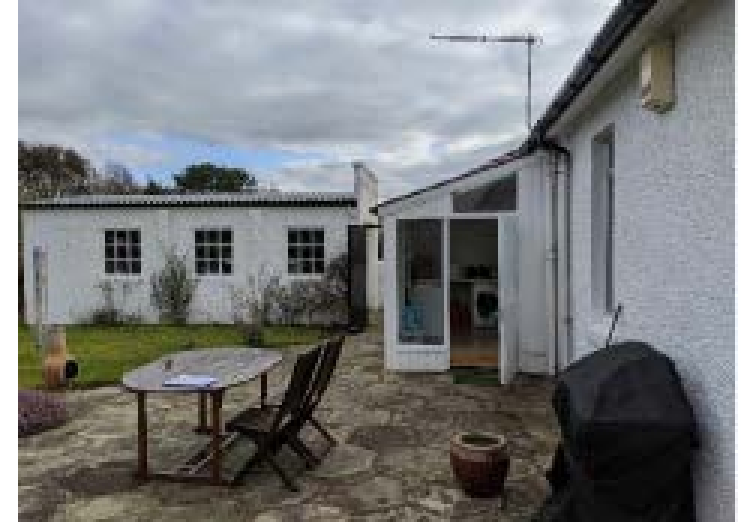
Part rear elevation showing existing garage
