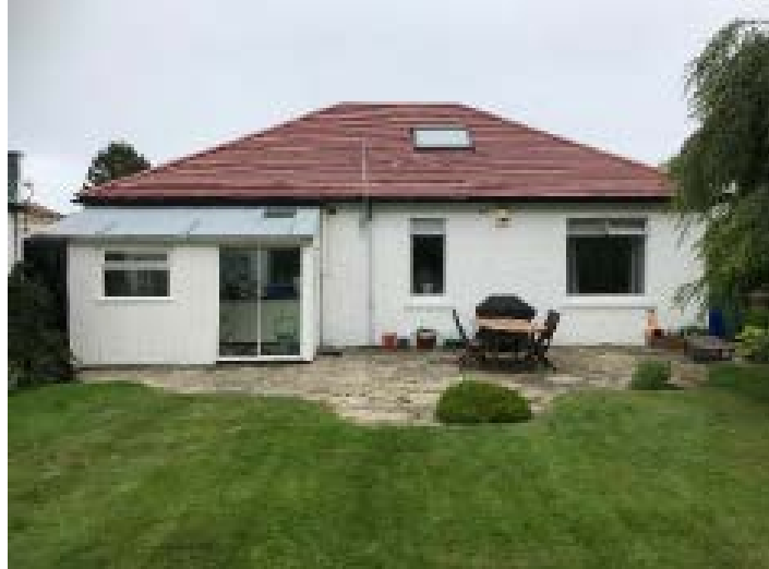
Rear elevation of existing property
