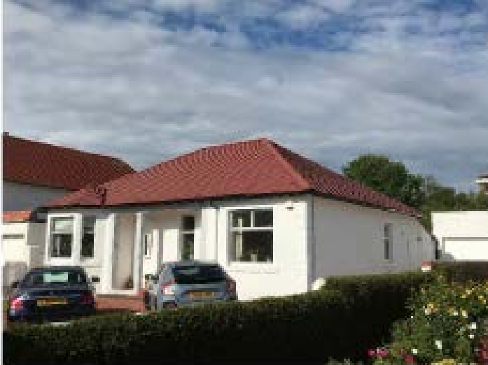
Principal elevation of existing property
