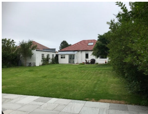
view from bottom of garden back to house including the garage
