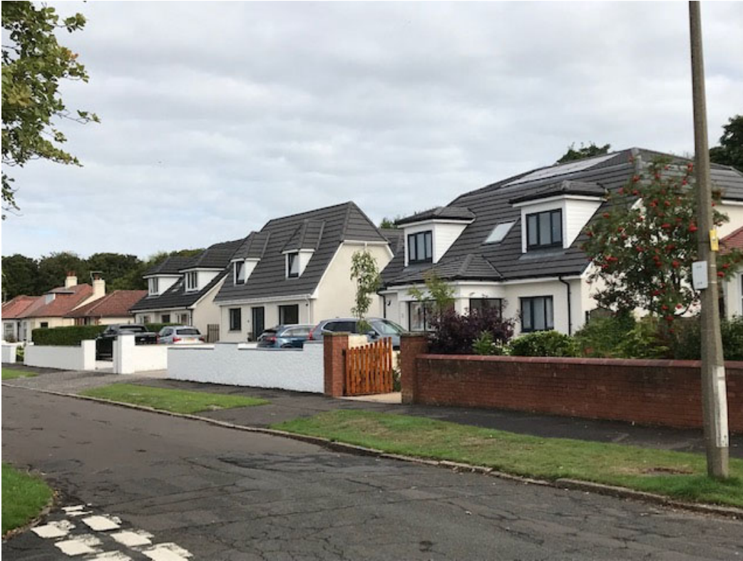
Streetscape further North at 16,17 & 18 Fullarton Crescent (18 nearest camera)
