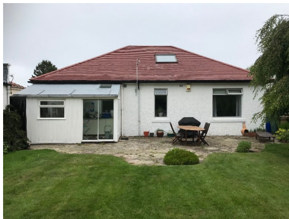
view to rear of dwelling
