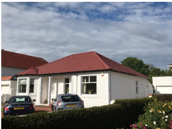
View from approach
