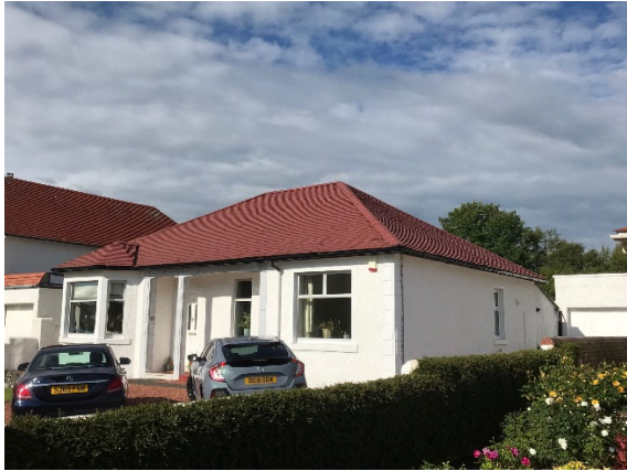
View from approach
