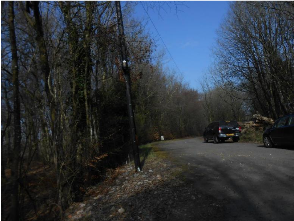
GENERAL VIEW ON SITE ENTRANCE – BT POLES AND OVERHEAD CABLES EVIDENT
