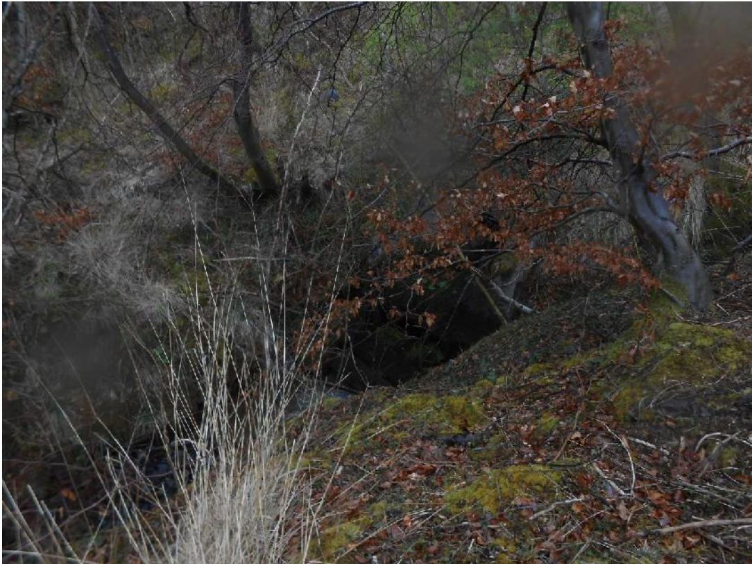
GENERAL VIEW ON STORM WATER OUTFALL – BEHIND TREE/BRANCHES - E236818, N618116
