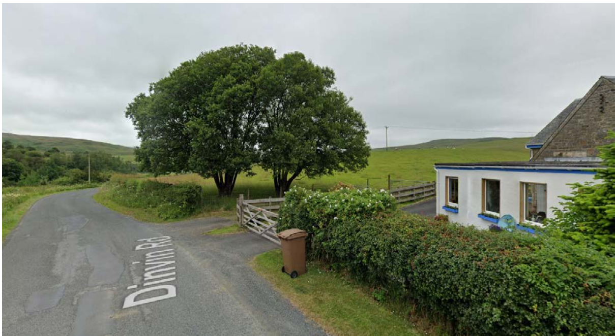
View of site from Dinvin Road to south (Google image)
