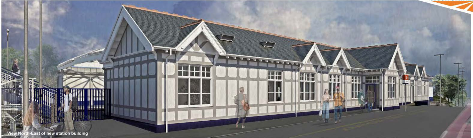
View North-East of new station building
