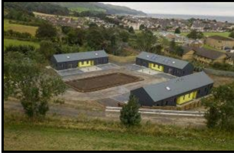
Houdston Reid Travelling Persons Site – Coalpotts Road Girvan, Finished Units
