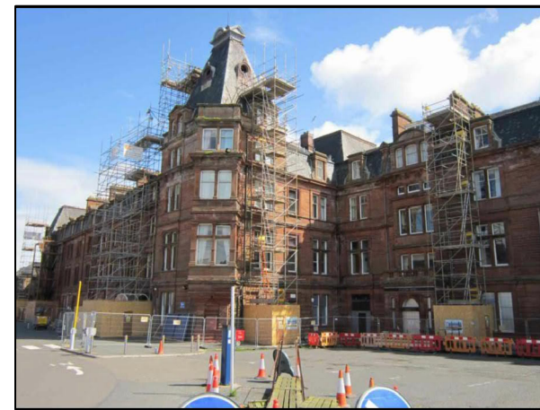
CLOCK TOWER PRIOR TO ENCAPSULATION INSTALLATION
