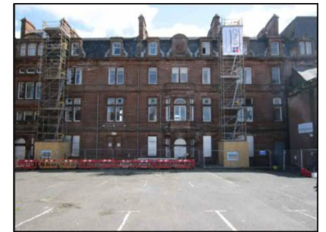
EAST ELEVATION PRIOR TO ENCAPSULATION INSTALLATION
