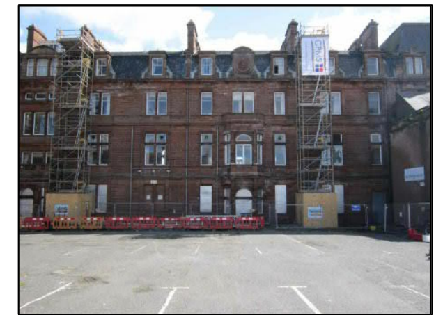
EAST ELEVATION PRIOR TO ENCAPSULATION INSTALLATION
