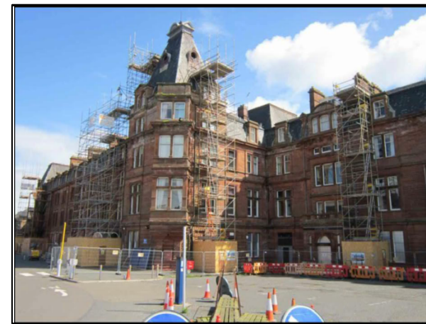
CLOCK TOWER PRIOR TO ENCAPSULATION INSTALLATION
