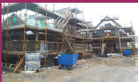
Progress photos: February 2024
