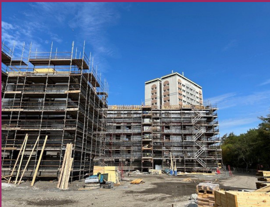
Progress at the Riverside
