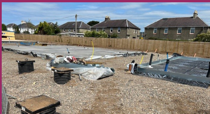
St Ninians New builds underway
