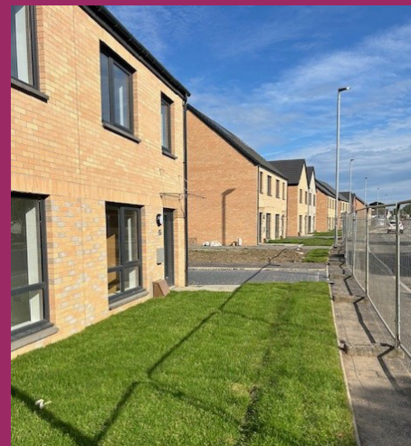
Mainholm New Builds
