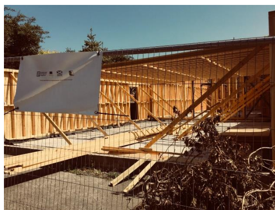
Figure 23: Dalry Scout Hall build project
