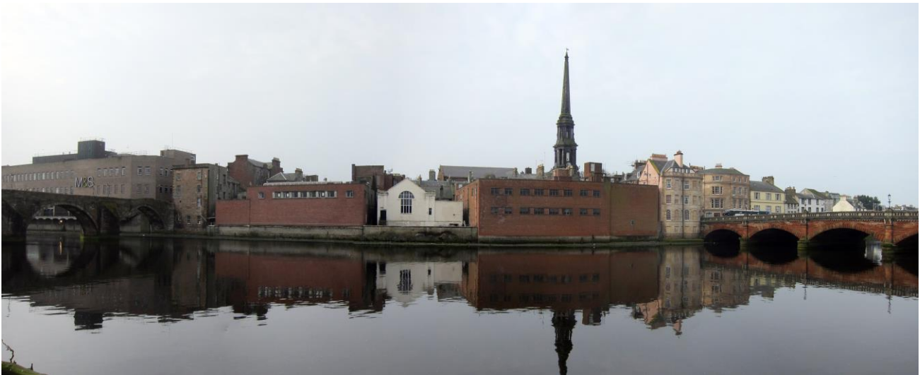
Ayr Riverside Block today. 20 th century redevelopment resulted long unrelieved 1930s brick elevations to the riverfront. The monolithic nature of these 1970s buildings is at odds with the medieval rig pattern and diversity of buildings in historic core of the town.
