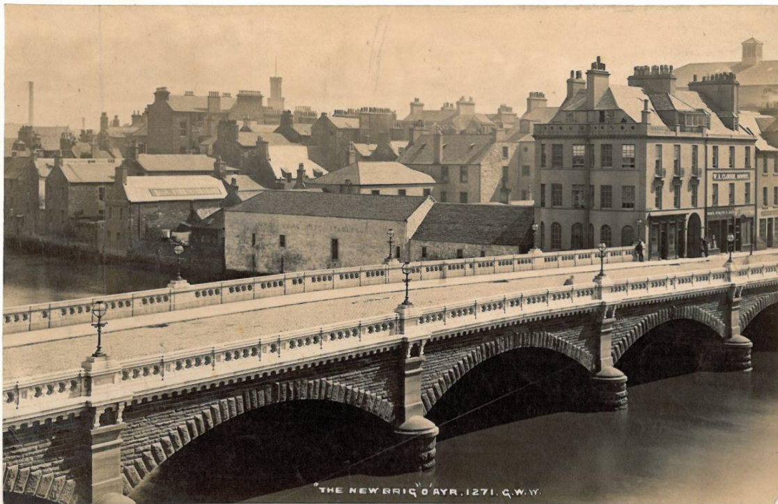
Early 20 th century photograph of the Riverside from east of the New Bridge. The diversity of building type and varied roofscape within the Riverside Block is evident.
