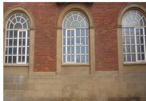
Metal-framed windows with a casement opening mechanism.
