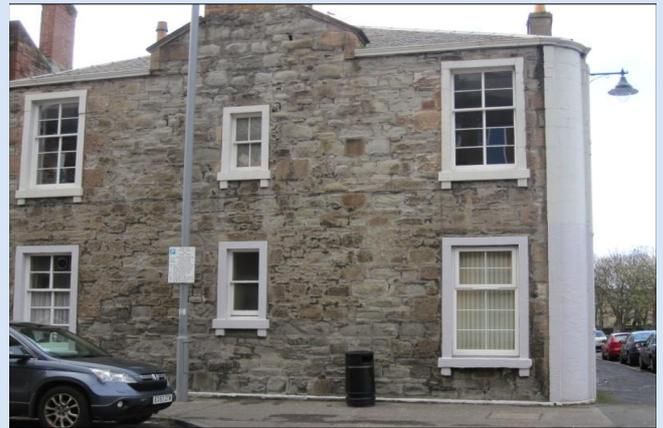
The character of this building has been adversely affected by the replacement window on the bottom right which uses uPVC, sandwiched astragals and a visible trickle vent.
