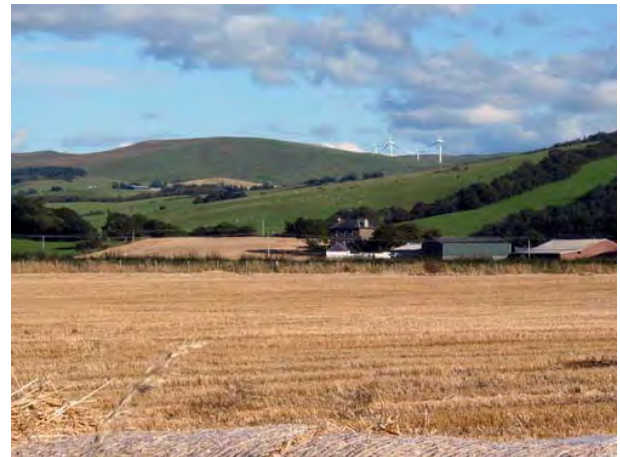
Hadyard Hill wind farm is located in a dip between the hills, which reduces its visual impact.
