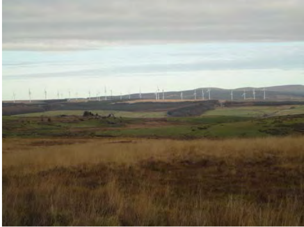
The operational Mark Hill wind farm sited on a simple 'platform' above the Duisk valley
