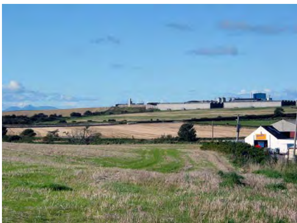
Larger sheds and buildings at the industrial site, including the distillery, are prominent on the skyline
