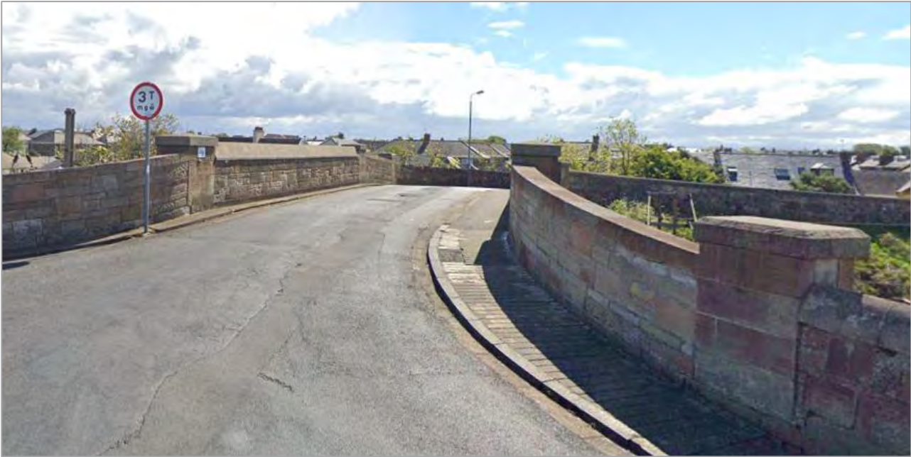
Figure 2-4: Bellrock Road – Weight restricted bridge (Source: Google StreetView)
