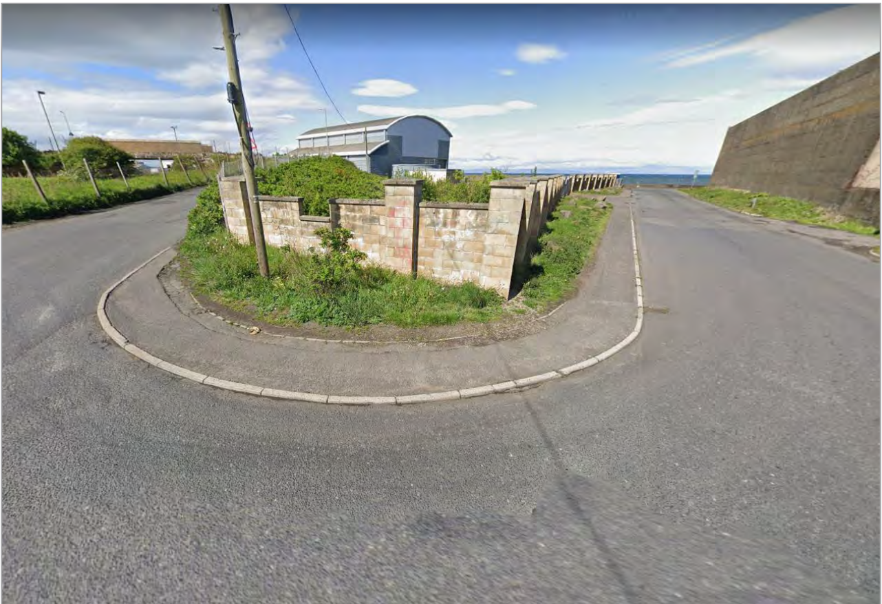
Figure 2-3: Saltpans Road – Hairpin turn (Source: Google StreetView)
