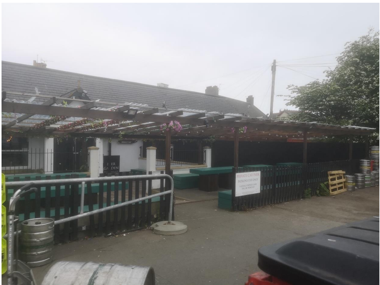
Photograph 1 – Showing the external drinking area as currently approved for permanent use
