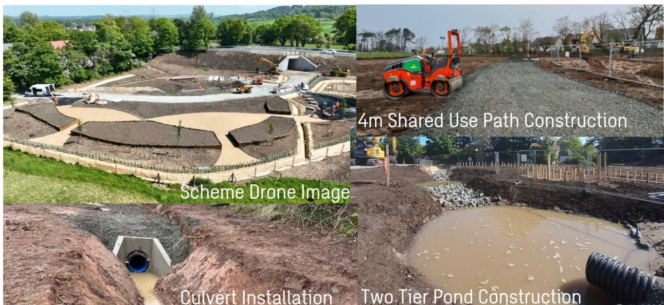
Figure 0-2 Photo collage showing different elements of the construction phase
